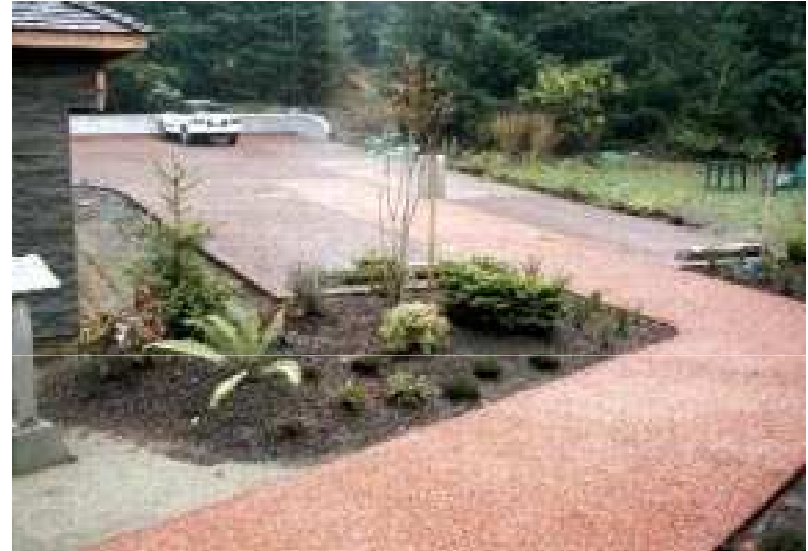
Colored pervious concrete walkway, Bainbridge Island, WA (G. McKinnon)
