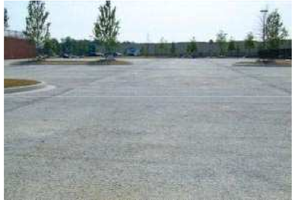
Large concrete parking lot, Buford, GA
