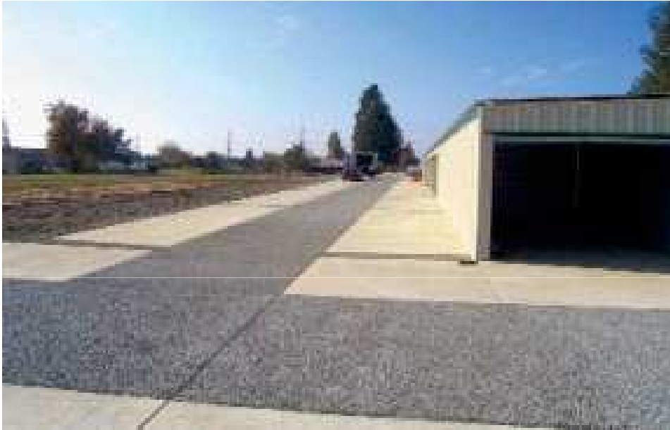
Storage facility lot, Mt. Angel, OR (R. Banka)
